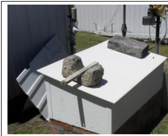
Outside view of vault
